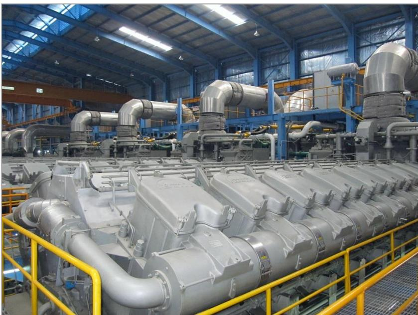
Four MAN 18V48/60TS engines generate electricity at the Belawan power plant.
